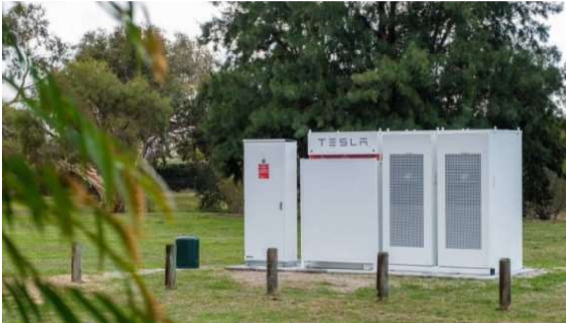
Figure 13 Powerbank installation in Western Australia
